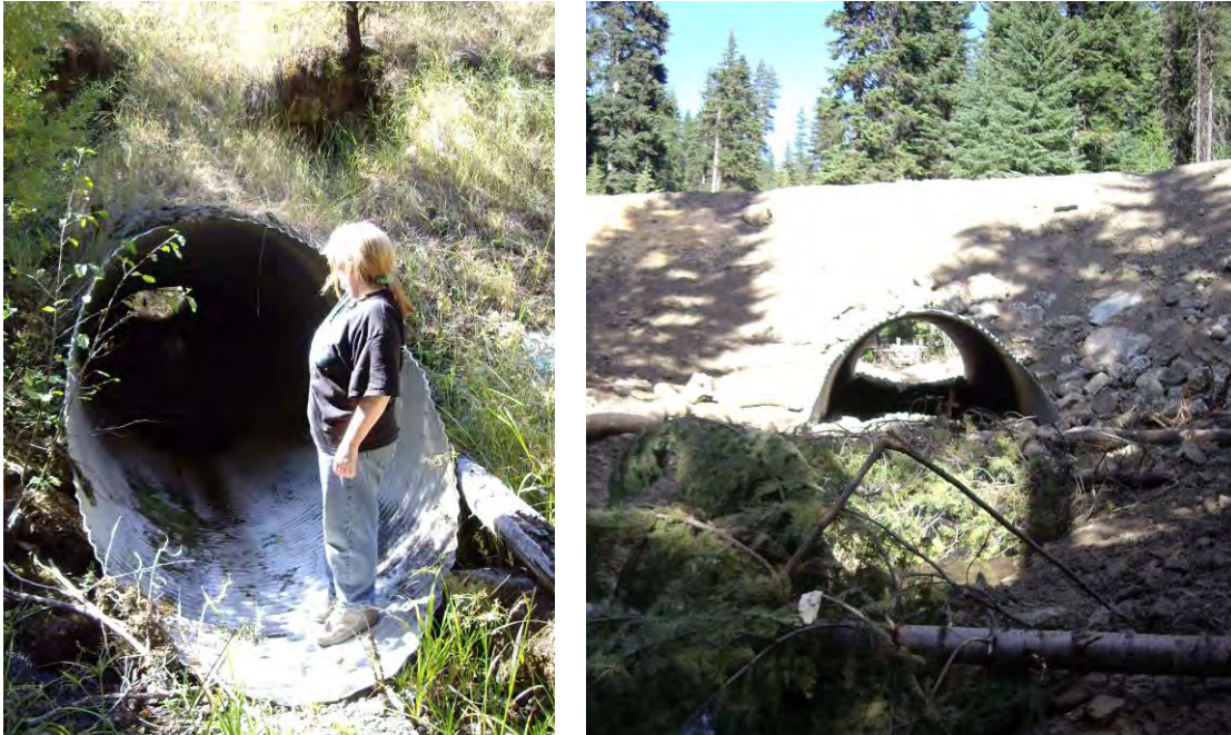
Figure IV. The Bruin Creek culvert before (left) and after (right) replacement. Note erosion above and around the old culvert and streamflows entering the culvert at the first seam.
