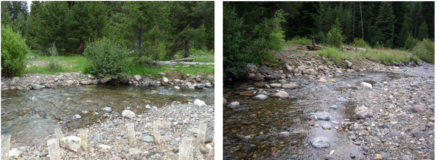
Figure VI. Scoured streambank in June of 2011 (left) and larger material placed during August of 2011 (right).
